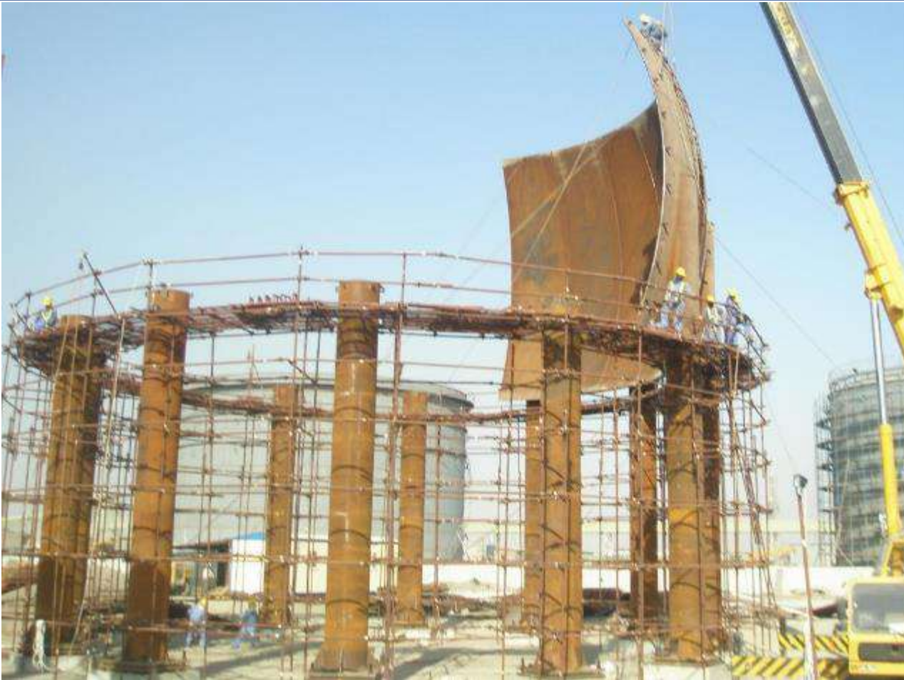
ERECTION OF SPHERE COLUMNS AND EQUATORIAL PETALS
